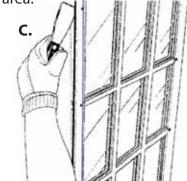
Carefully remove any residue on the door and prepare the surface for your new door lite. Use a putty knife to help remove any dirt, excess caulking or paint, and clean the surface using window cleaner and towel on both sides of the opening. \*Note: the edge of the door can be sharp. Please take caution when cleaning around this area.
