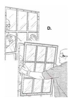
Install your new Trimlite door lite. Remove the inner frame (the side with screw holes) of your new door lite and set close by inside. Have one person (D.) lift the exterior frame and glass into position from the outside. Set the new glass into the bottom edge of the opening. Using one hand, maintain pressure keeping the frame in contact with the bottom edge of the door opening.
